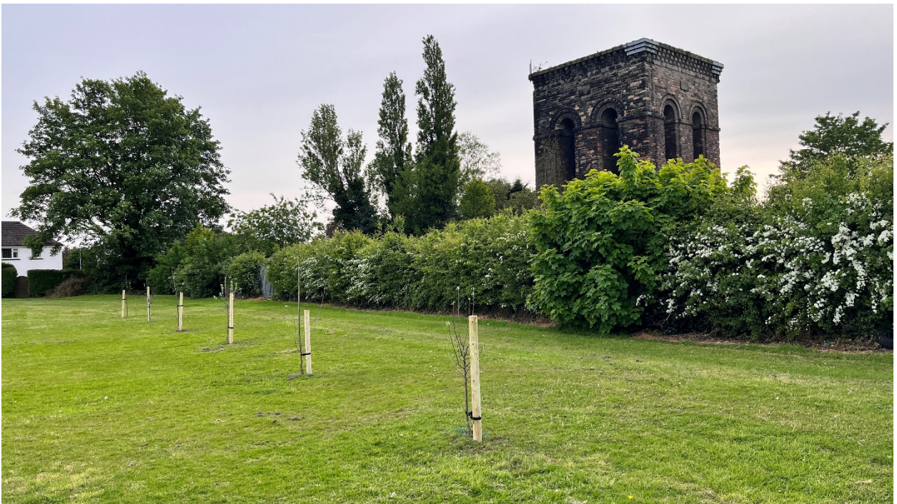
Tower Hill, Ormskirk
